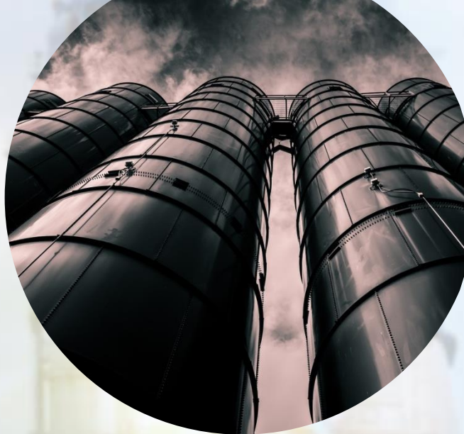
Silos D= 11,5m H= 13m
