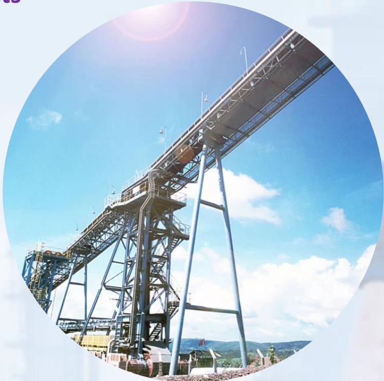
Transport conveyors up to 130m length
