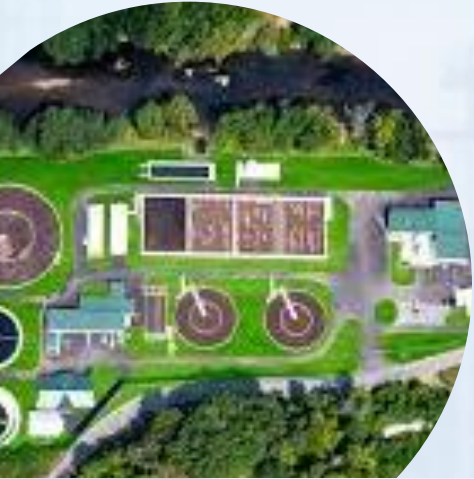
Wastewater treatment plant 2 500 m 2
