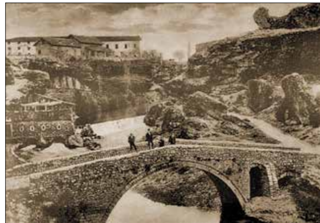
Ribnica Bridge (Most na Ribnici)
